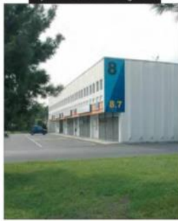
Capannone Isola 8 - Building Area 8
