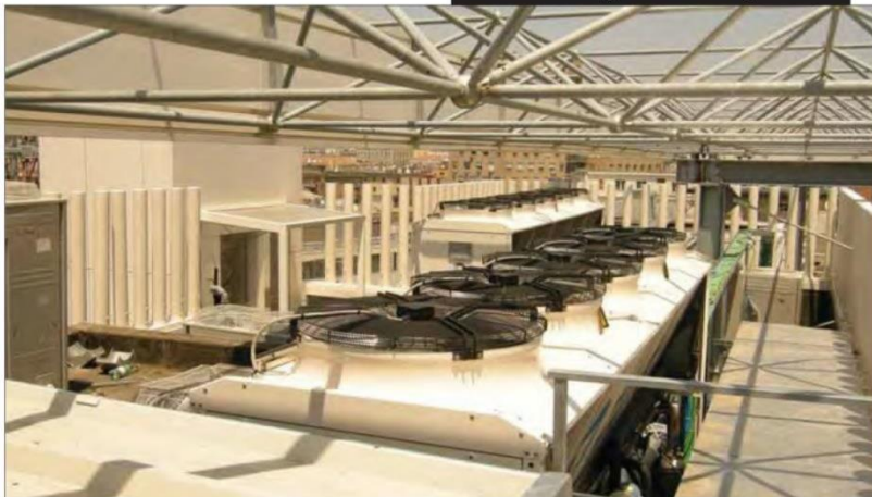
Centrali tecnologiche - Technological station
